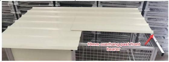
4. Ensure the front and rear sheets align and centre the sheets to have equal overhang each side, rechecking for a 10mm overhang on the front and being aligned through the sheet overlaps sections.
