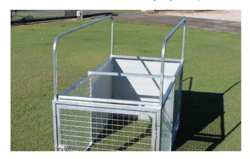
Recheck diagonal measurements are still equal. If they are not, adjust until unit is square. Then tighten all bolts firmly.
