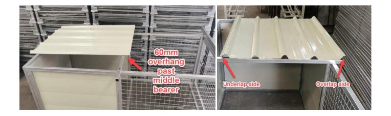
2. Then place the next sheet to overlap the first sheet, ensuring the overlap side of the sheet is on top of the first sheet. Centre the sheets on the kennel, ensuring equal overhang each side.
