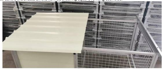
3. Starting from the same side as the rear sheets, place the first front sheet **ON TOP** of the rear sheets, ensuring the overlap side is facing out (same as the rear sheets). Allow a 10mm overhang at the front bearer. Repeat the process for the next sheet in the same sequence as the rear sheets.
