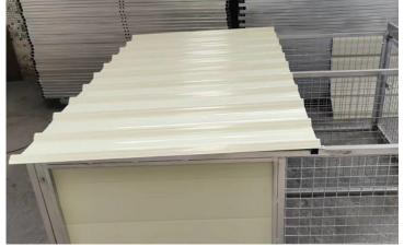
3. Starting from the same side as the rear sheets, place the first front sheet **ON TOP** of the rear sheets, ensuring the overlap side is facing out (same as the rear sheets). Allow a 10mm overhang at the front bearer. Repeat the process for the next 2 sheets in the same sequence as the rear sheets.
