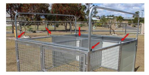
Recheck diagonal measurements are still equal. If they are not, adjust until unit is square. Then tighten all bolts firmly.
