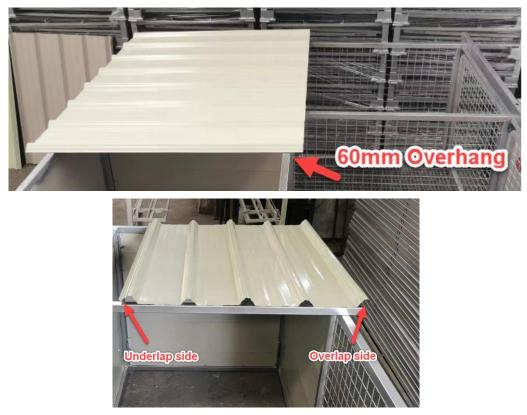
Place the next sheet to overlap the last sheet, ensuring the overlap side of the sheet is on top of the first sheet. Repeat with the third sheet and adjust the amount of overlap to centre the sheets on the kennel, ensuring equal overhang each side that the roof section is square with the kennel and there is 60mm overhang past the middle bearer.
