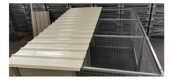
3. Starting from the same side as the rear sheets, place the first front sheet **ON TOP** of the rear sheets, ensuring the overlap side is facing out (same as the rear sheets). Allow a 10mm overhang at the front bearer. Repeat the process for the front row of sheets in the same sequence as the rear sheets.
